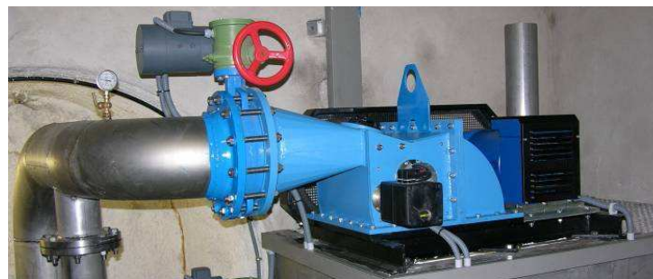
Microturbina BANKI-MICHELL
